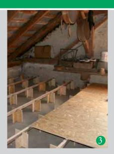
Lay the floor boards and fix them. With an 18 mm OSB wood-based panel, the construction is an accessible system with a very high load capacity.
