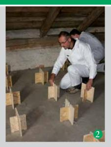
Set up the modules at a centre-centre distance of approx. 80 cm. Then place the 4/6 laths into the cut-outs provided (without screwing).
