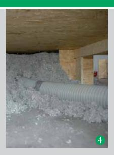
Afterwards the construction is filled with the ISOCELL cellulose.
