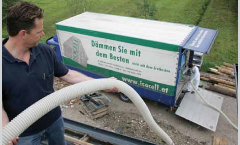
Only the injection hose needs to be brought to the place of installation, not enormous amounts of material.
